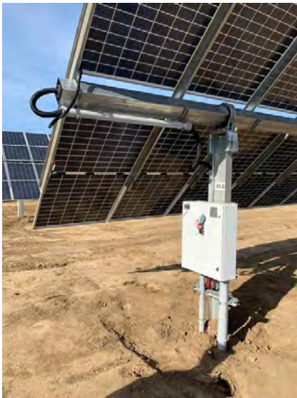
Single-axis tracker (Madison Gas and Electric Dane County Regional Airport Madison, Wisconsin, USA)
